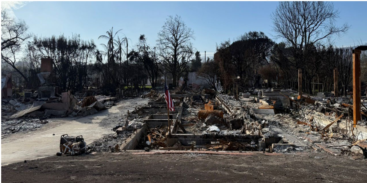
Photo information: Palisades Village. 2025 Palisades Fire. Photo credit: Erica Fischer
