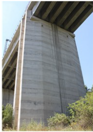
11 High-Speed Railway Viaducts (126 spans)
