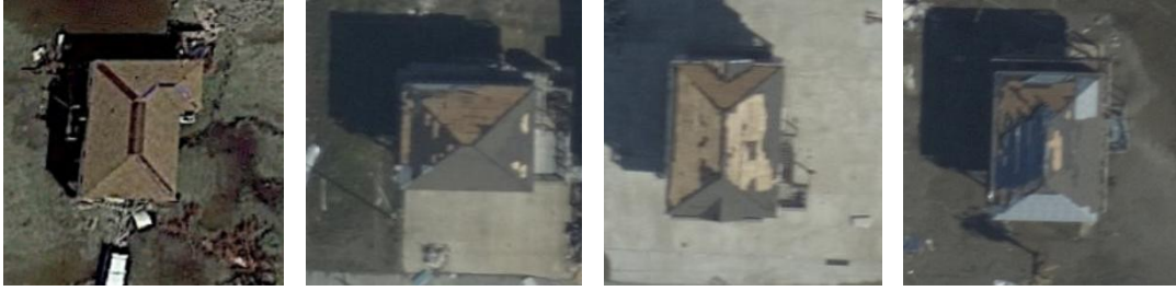
Figure 6. Examples of each roof cover damage state. From left to right: \leq 25\% damaged, >25\text{-}50\% damaged, >50\text{-}75\% damaged, >75\% damaged. Imagery obtained from NOAA aerial imagery.
