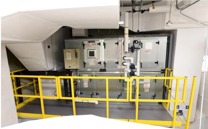
**Fig. 6. Picture of the OAU. Air is drawn in from the lower left, exits the OAU on the upper left of the unit, and goes to the AHUs at the right (not shown).**
