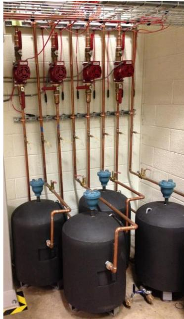
**Fig. 13.** The black tanks hold water for the thermal mass coils in the zone simulators. Above the tanks are the red circulating pumps that move the water through the TMCs. The flow rate is determined by manually setting a valve.
