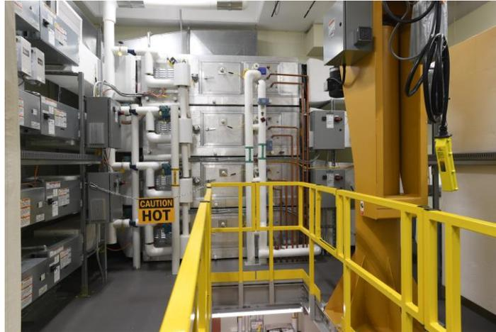
Fig. 12. Picture of the four ZSs. The VAVs are at the left.
