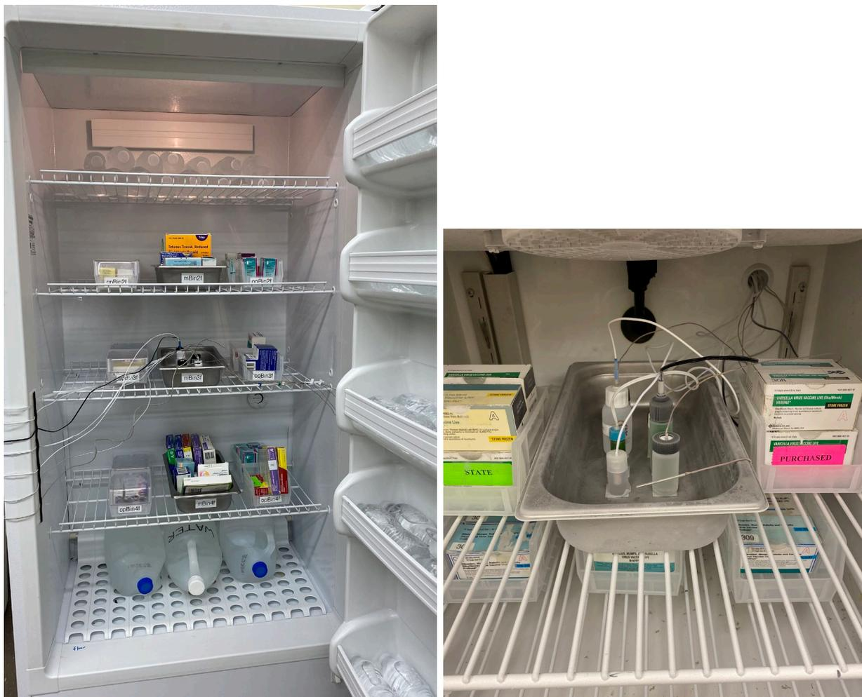
**Fig. 7a, 7b.** DDL installation in a standalone refrigerator (left) and an undercounter freezer (right).
