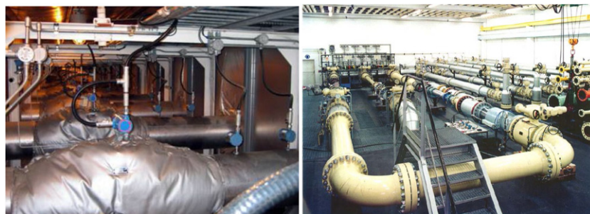
Figure 44. Working standard turbine meters used in parallel for natural gas flow measurement at (left) CEESI in Iowa. Reproduced with permission from [128] and (right) Pigsar in Germany. Reproduced with permission from [131].
