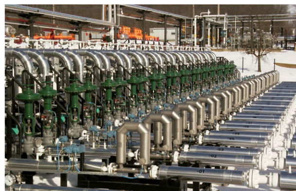
Figure 46. Twenty-seven Coriolis meters used in parallel at a natural gas storage facility in Hungary. Reproduced with permission from [138]. Photo courtesy of Emerson Automation Solutions.
