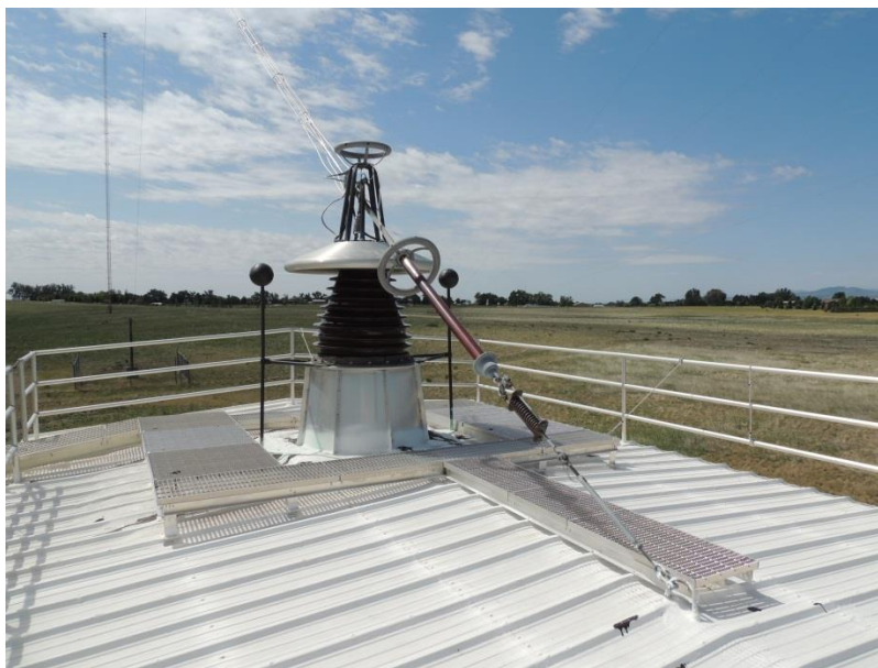
Fig. III.A.8. Roof of helix house and connection to antenna array.
