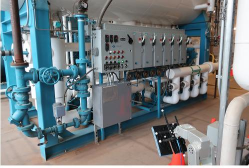
Fig. 3. Data collection in the NIST Central Utility Plant (CUP). The receive antenna is shown at lower right. It is located in front of a piece of RF absorber and mounted to a robot arm that scans to form the synthetic aperture array. The same measured data was used in assessing the initial version of the proposed approach in [34].
