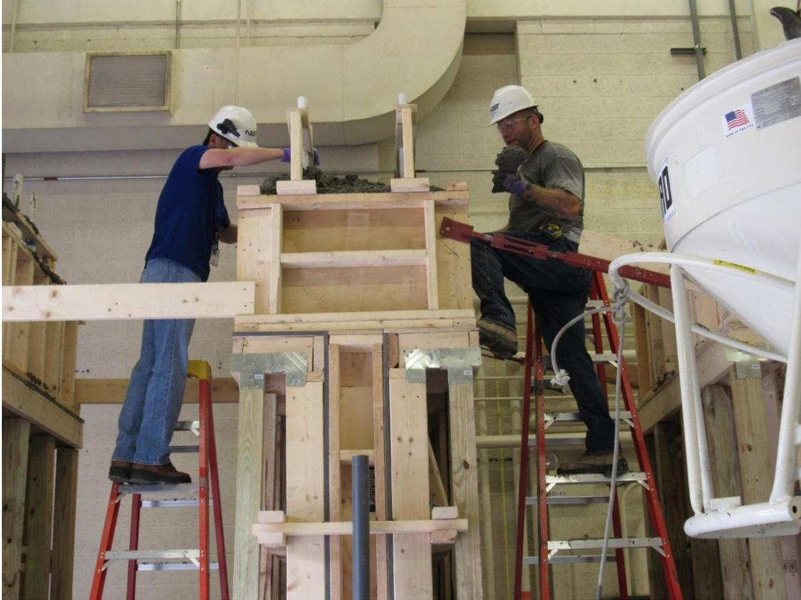
**Figure 2.13: Concrete placement into the top cap formwork and consolidation using vibrators.**
