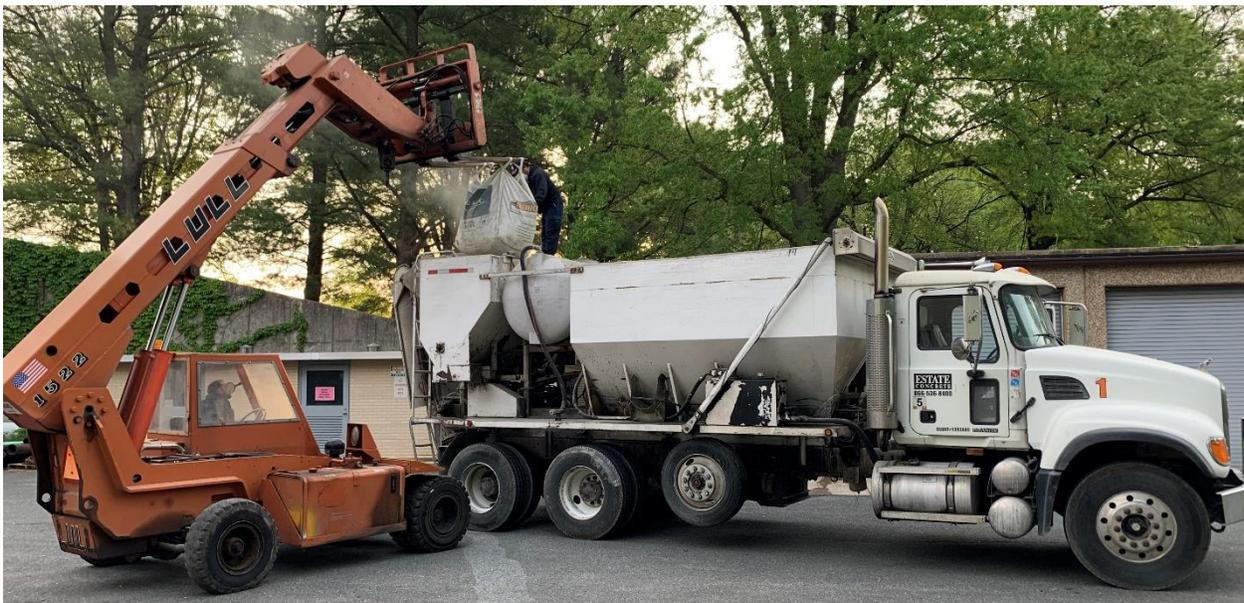
Figure 2.9: Loading of aggregates into volumetric truck mixer
