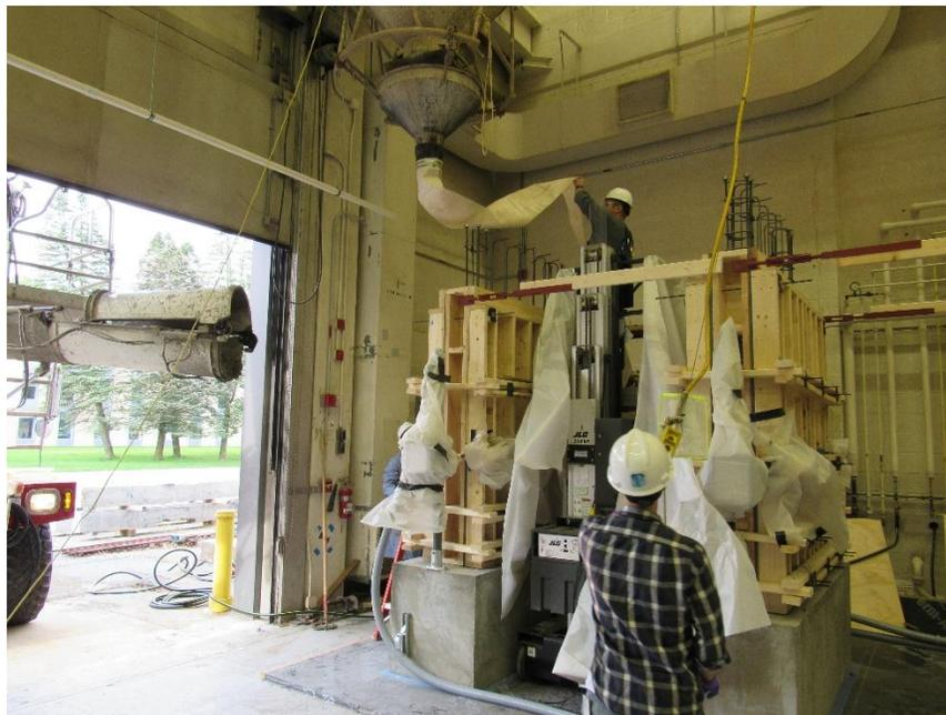
**Figure 2.11: Concrete placement into wall's formwork and consolidation using vibrators**
