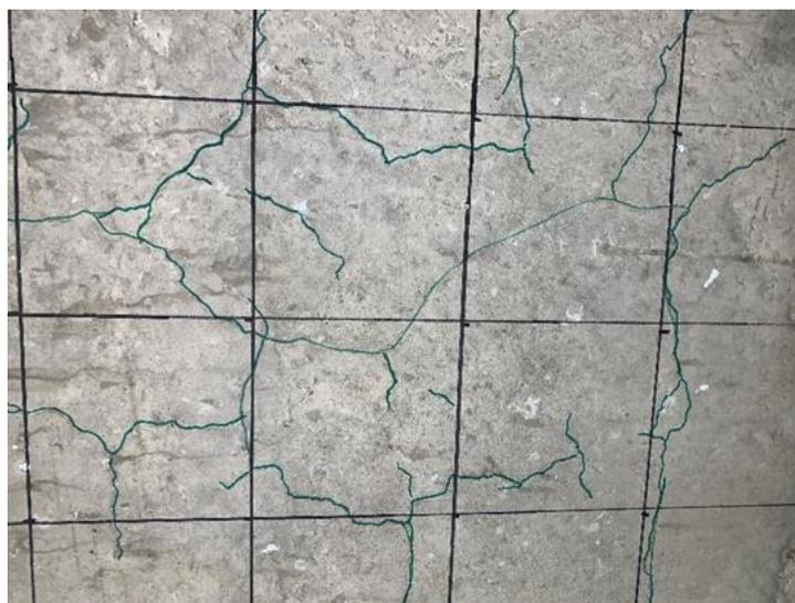
**Figure 3.2. Exudation of a white substance on the face of reactive walls. Cracks highlighted using permanent marker.**
