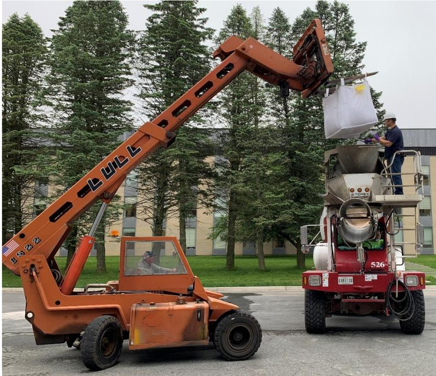
**Figure 2.12: Loading of aggregates into concrete mixer truck**
