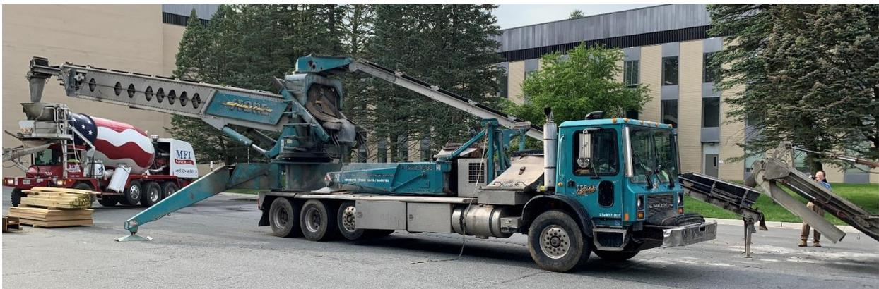
Figure 2.10: Loading the volumetric truck contents to a concrete mixer truck via a conveyer belt (telebelt)
