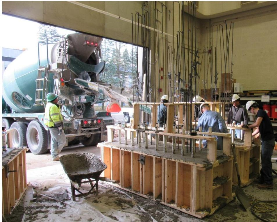
**Figure 2.8: Concrete placement into the footings formwork and consolidation using vibrators**
