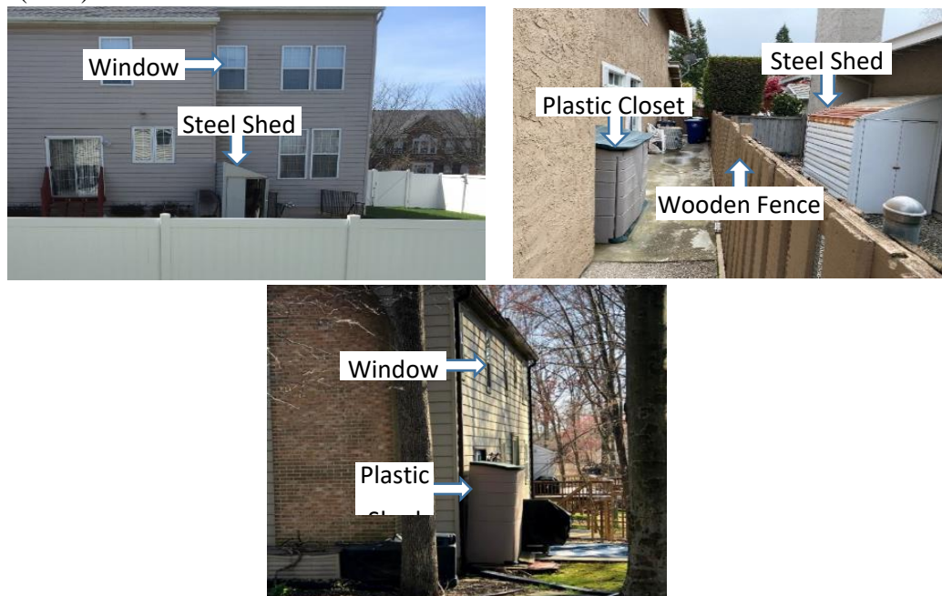
Figure 1: Photos of very small and small sheds in common locations against the primary structure and near additional vulnerabilities such as windows and combustible fencing. Photo Credits: NIST.
