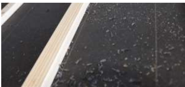
Figure 3 Battens and underlayment after the time have been removed. Applied wind speed of 6 m/s and 2 kg of water was applied before an experiment.
