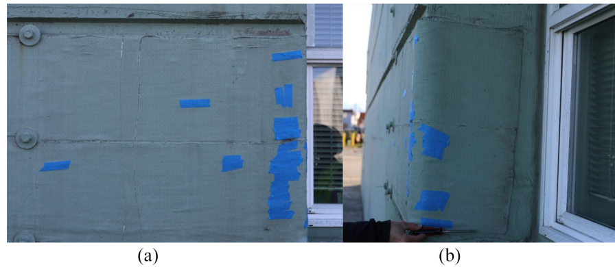
Figure 14. Exterior CFRP retrofits at MKT: (a) One area and (b) a collected CFRP sample from CFRP locations with poor epoxy saturation and (c and d) areas where moisture or water was present.
