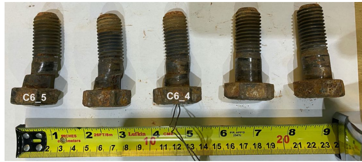
Figure 13. Post-fire inspection on the bolts from connection C6.
