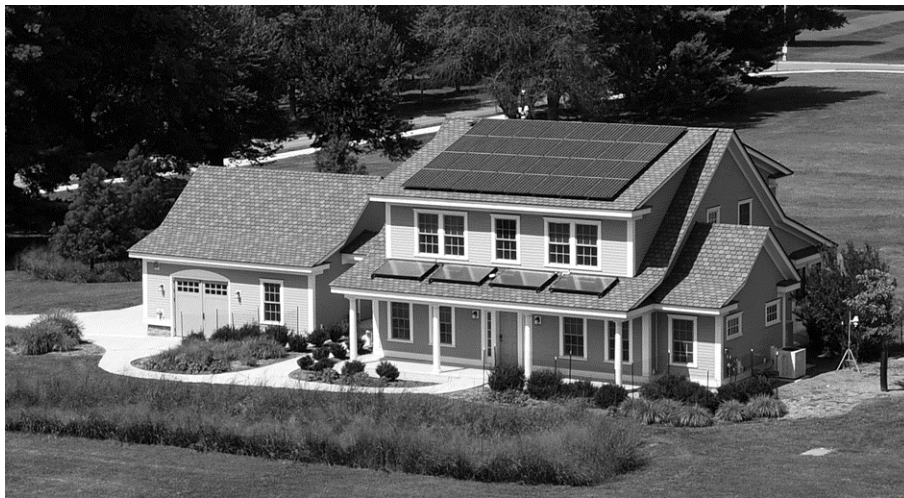
Figure 1: NZERTF south view
