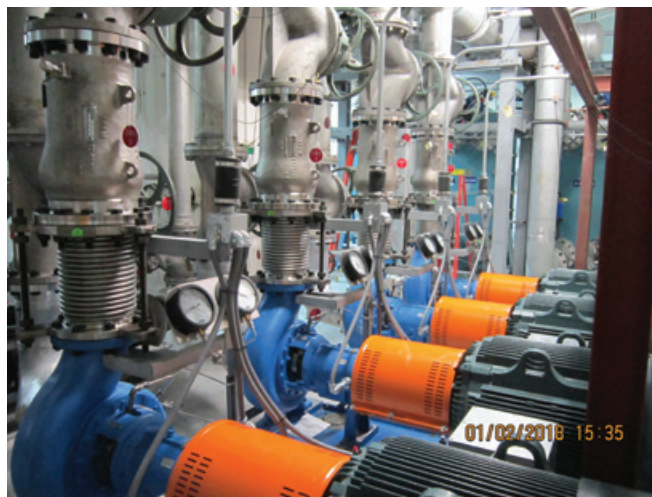
FIGURE 7: New primary cooling pump assemblies. The new pumps are physically larger than the old pumps and as a result run cold to the touch, while the old pumps operated at ~ 45 °C. What appear to be stainless-steel spool pieces (with the lifting lugs) are in fact the new nozzle check valves, which operate on flow (or lack thereof) alone as opposed to the old check valves, which operated on external air pressure.
