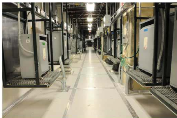
Fig. 2. Interior of basement level in Building 1
