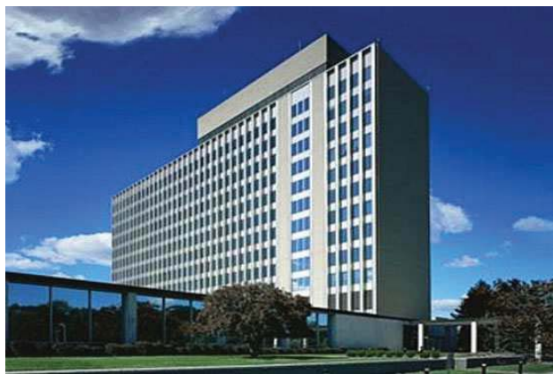
Fig. 6. The building used for the live tests
