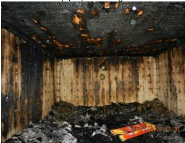
(c) interior with gypsum board removed
