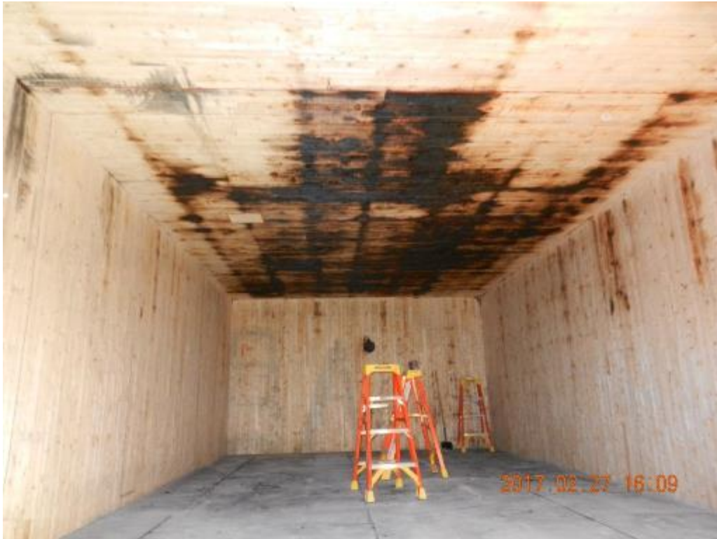
(a) CLT structure after repair
