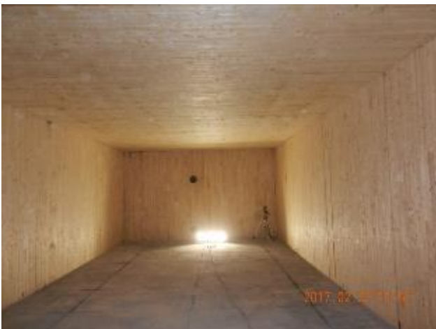
(g) after cleanup and removal of gypsum board
