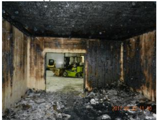
(d) interior with gypsum board removed
