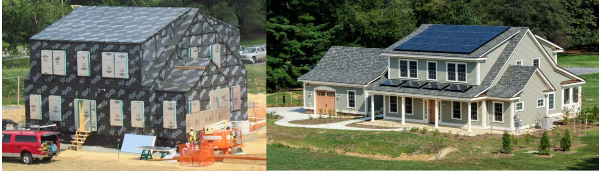
Figure 1. Left: continuous air barrier system. Right: NZERTF upon completion.
