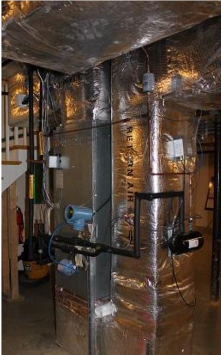
Figure 3. Instrumented Air-to-Air Heat Pump Interior Unit with Dedicated Dehumidification Cycle.
