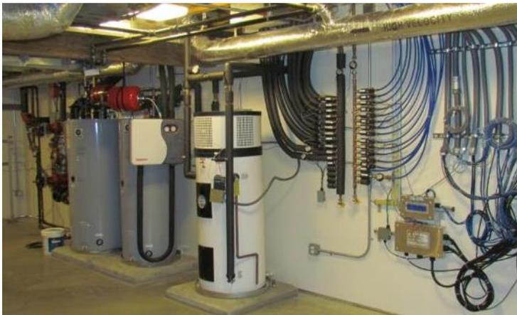
Figure 4: Two-tank solar and heat pump water heater system with distribution manifold system. Second solar storage tank on left is reserved for future studies.
