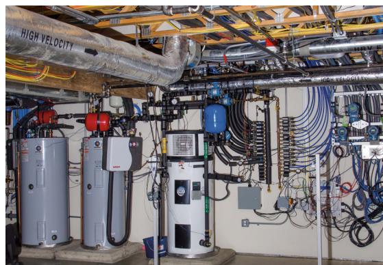
Basement of NZERTF showing ductwork, water distribution system, solar hot water storage tanks, heat pump water heater, and associated instrumentation.
