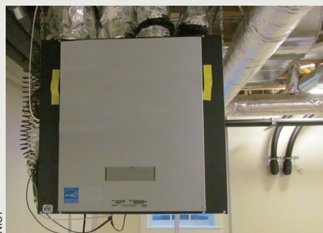
A heat recovery ventilator is used to condition outdoor ventilation air prior to it being introduced into the NZERTF. The HRV exchanges thermal energy between the entering and exiting ventilation air.
