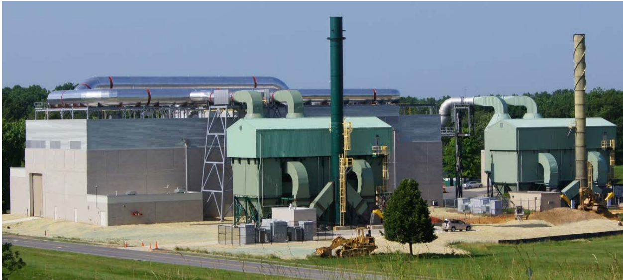
Figure 9 The National Fire Research Laboratory (NFRL). CO 2 emissions are predicted using fuel consumption measurements for natural gas. The predicted CO 2 emissions are used to quantify the accuracy of CEMS and RATA measurements in the rooftop exhaust ducts. ( http://www.nist.gov/el/fire_research/nfrl.cfm )
