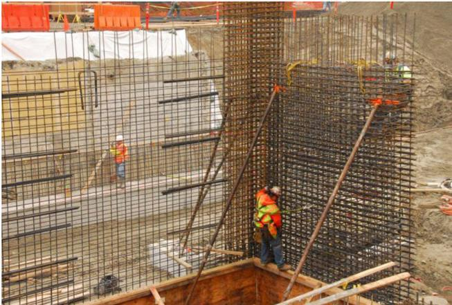
Figure 7-3 – Boundary confinement for wall flange.
