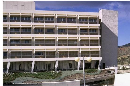
**Figure 2-4** – Weak story damage, 1971 San Fernando earthquake.
