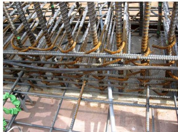
**Figure 7-2** – Boundary confinement for planar wall.
