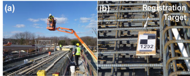
Figure 2: (a) data collection; (b) registration targets
