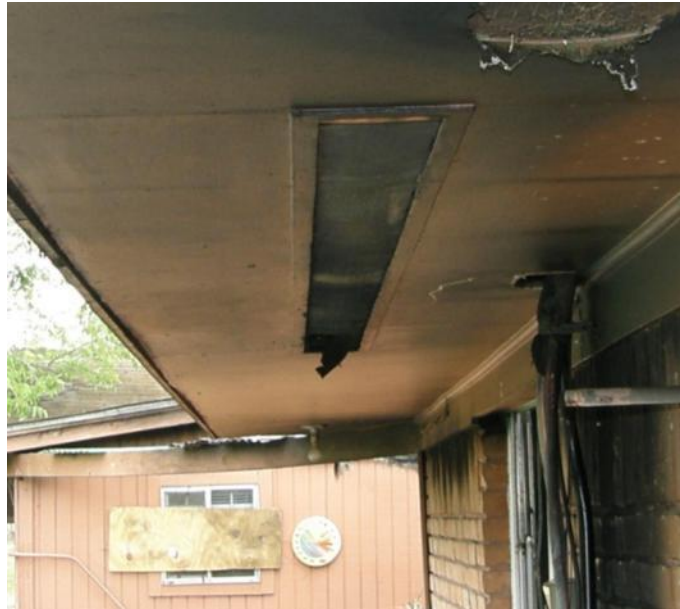
Figure 12: Soffit vent on the B-side (North) of the structure
