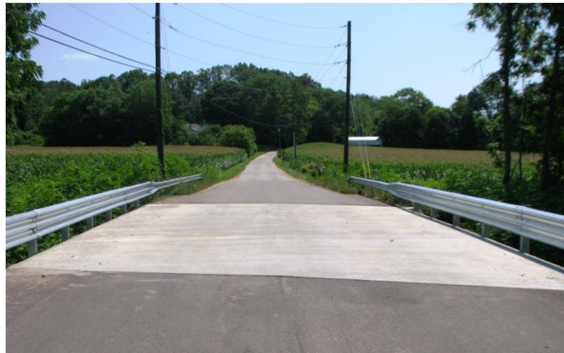
Fig. 3. Currently “crack free” internally-cured concrete bridge deck in Monroe County, Indiana after 1 year in service.
