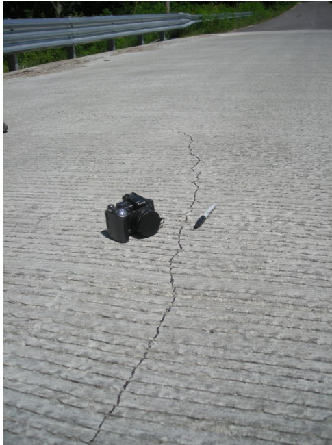
Fig. 2. Cracking that occurred when using a “conventional bridge deck mixture” in Monroe County, Indiana.
