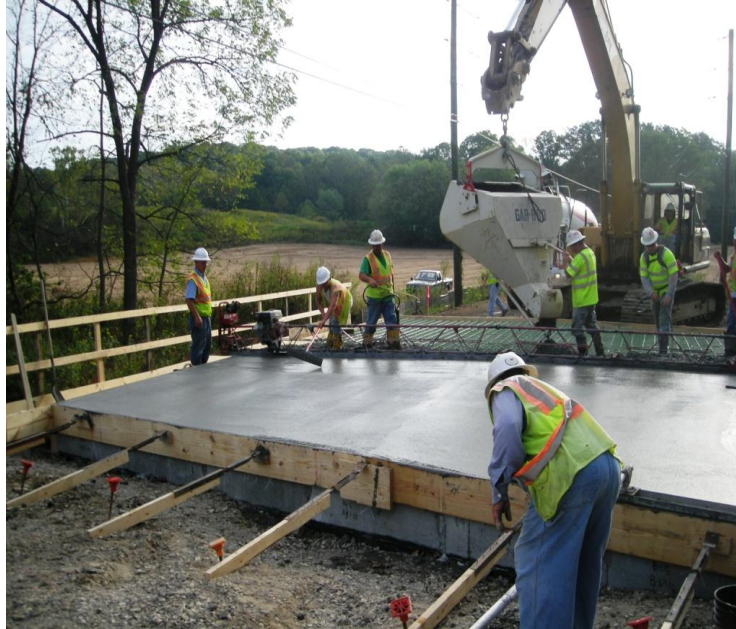
Internally-cured concrete being cast in a bridge deck, Monroe County, Indiana.
