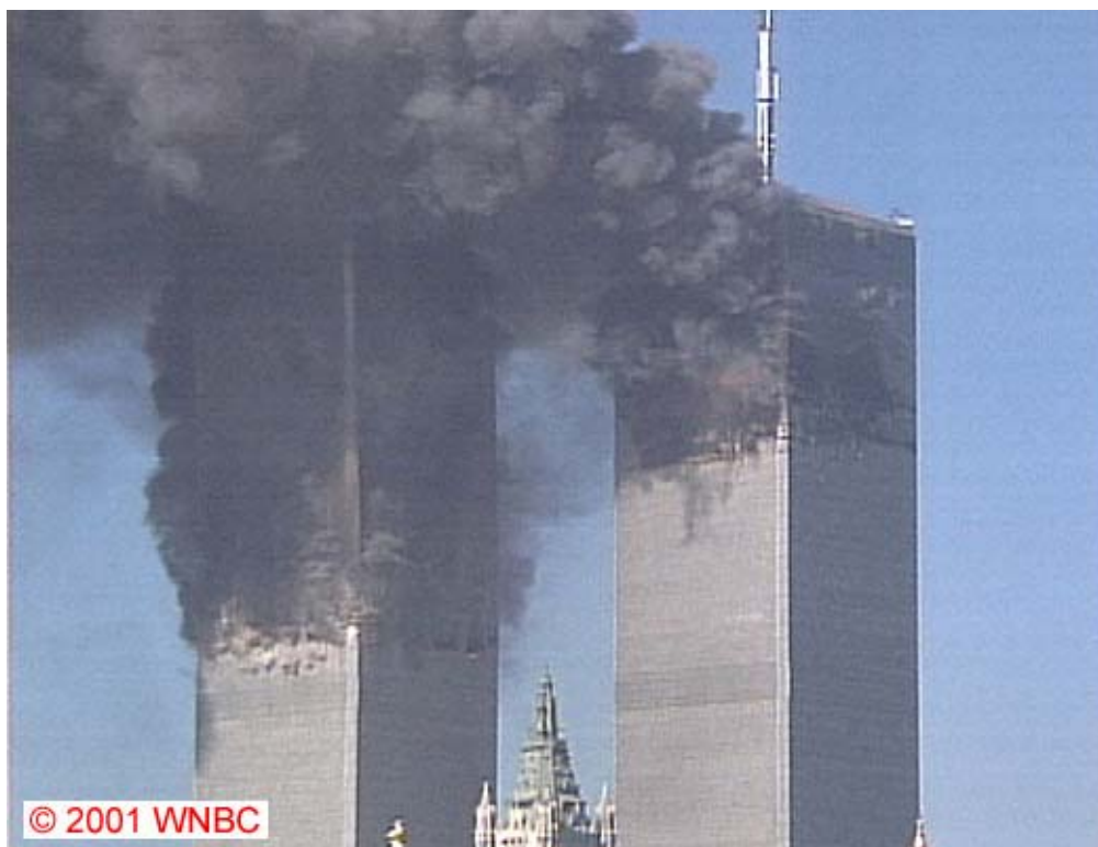
Figure E-16. Initiation of collapse of WTC 2. Note the tilt toward east and south.
