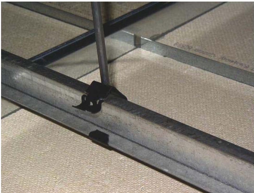
Figure 2–17. Bottom CADDY fastener in suspension system 1.
