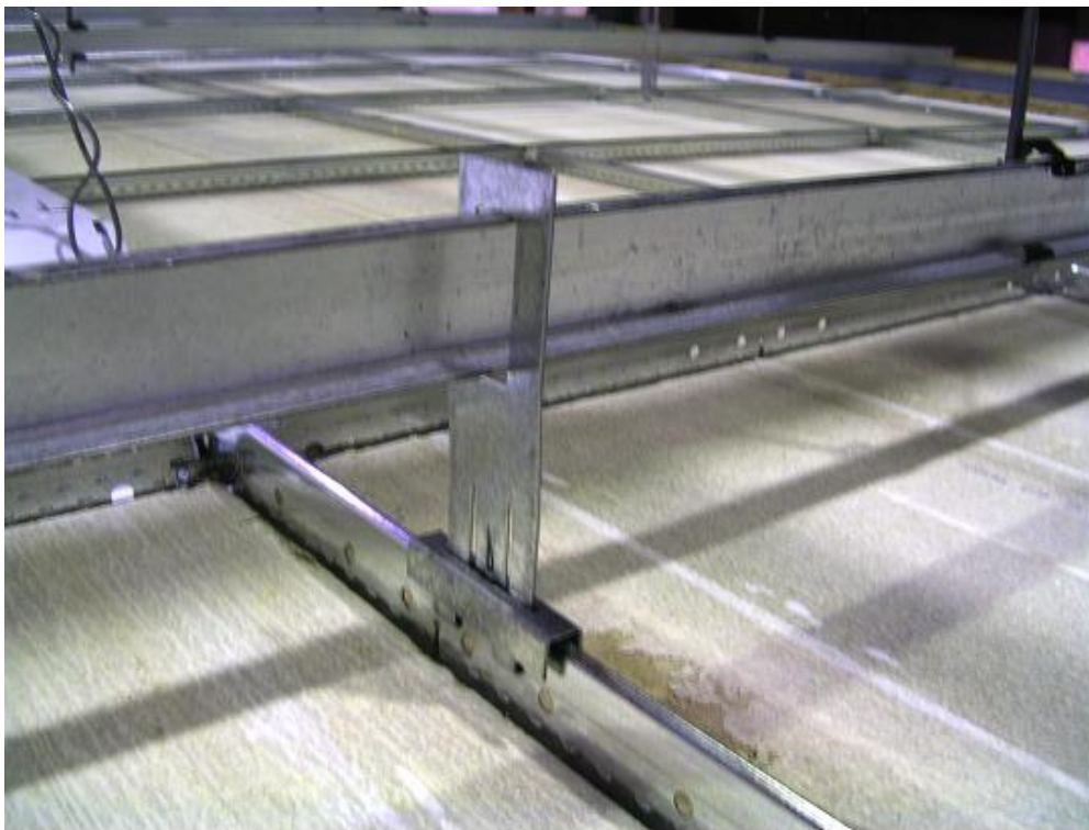
Figure 2–24. CBS clip connecting channel to main runner in suspension system 2.
