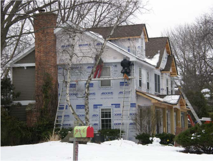
Figure 1. Modern houses use plastic sealing wrap to exclude water and multi-pane windows to improve energy efficiency.
