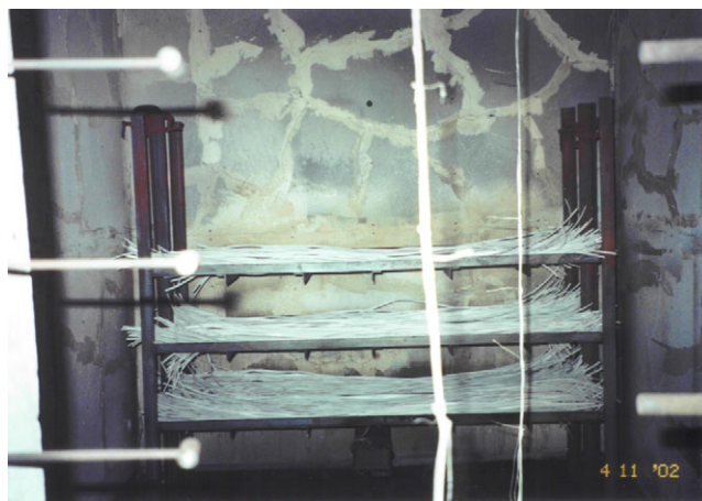
Figure 7. Photograph of cable trays in the burn room.
