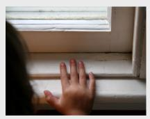
Deteriorating paint on window sills can get on the hands of children and be ingested, increasing the likelihood of lead poisoning if it's an older home.
