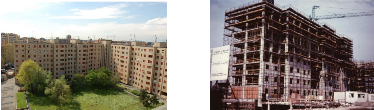
Figure 3. District Via Giuffrè/Villani, Milan: example of prefabricated building.
