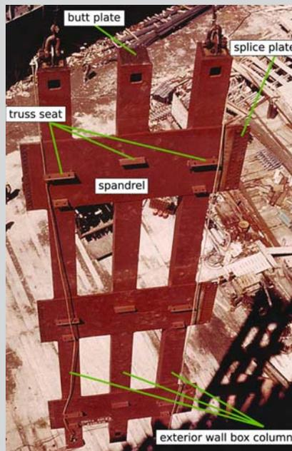
Figure A. Images of the exterior wall columns and floor truss assemblies during construction of the towers. The figure shows the major structural components and how they were assembled (Source unknown).
