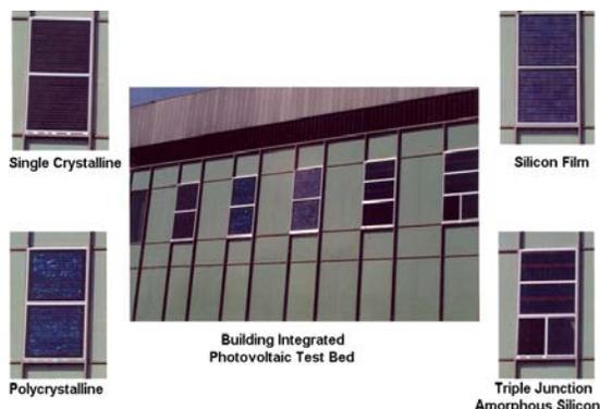
Figure 1 Photovoltaic BIPV Test Bed
