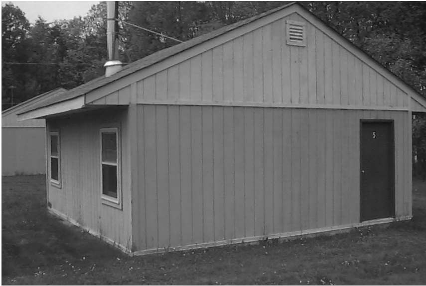
Figure 2. Single zone test house
