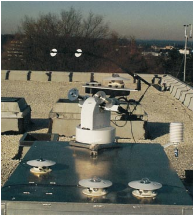
Fig. 7 Rooftop meteorological station
