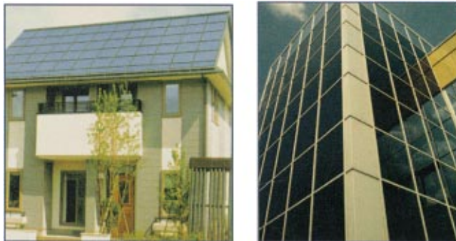
Fig. 2 Building integrated photovoltaic examples (Source, Paul Maycock)
