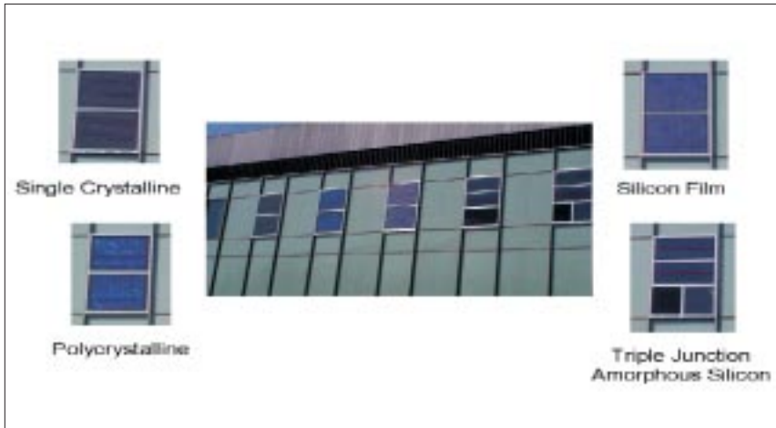
NIST's Building Integrated Photovoltaic Test Bed.
