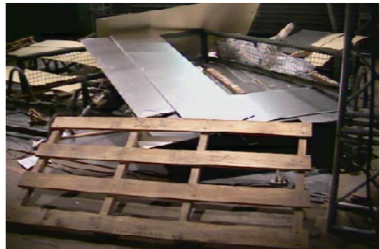
Figure 4b: Collapsed housing materials in the MeSci Red arena
