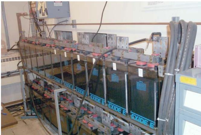
Figure 3. Subsecond Thermophysics Laboratory power supply. FET switches are located at top left.
