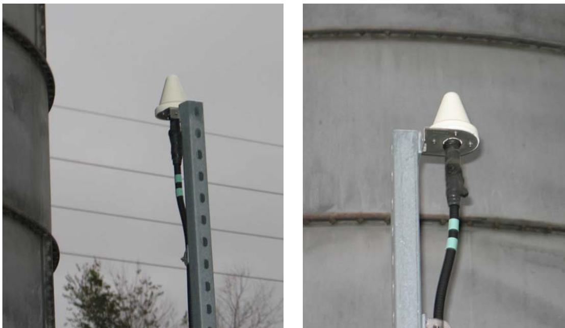
*Figure 4. A GPS antenna at a CDMA base station with an obstructed view of the sky.*
