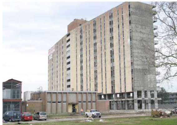
Figure 1: New Orleans apartment building.
