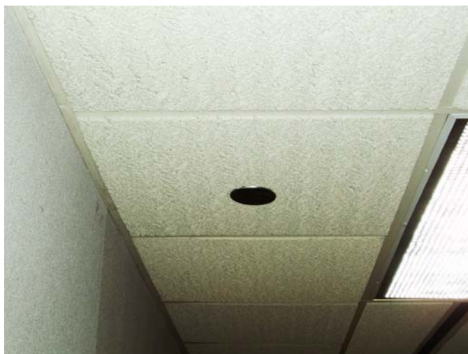
Figure 5–10. Typical concealed pendent sprinkler.
