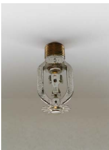
Figure 5–11. Typical standard spray pendent sprinkler.
