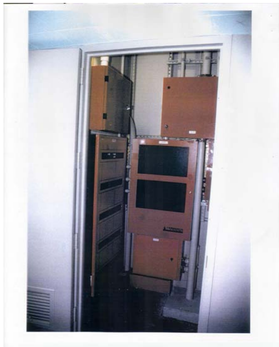
Figure 5–19. Fire alarm closet with PSR location.
