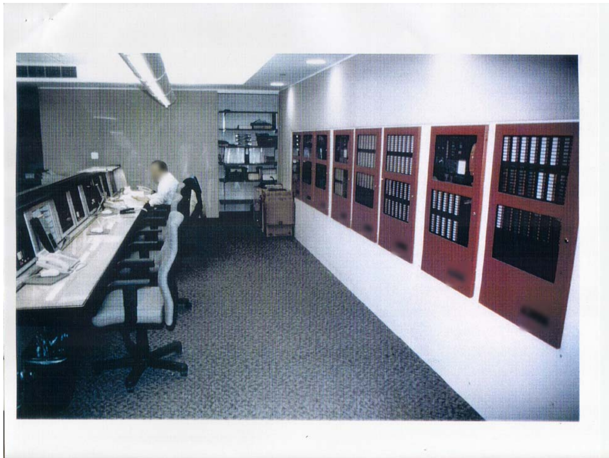
Figure 5–25. Operation Control Center located on the B1 Level below WTC 2 with redundant fire alarm system controls.
